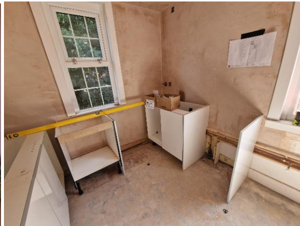
New main kitchen units going in
