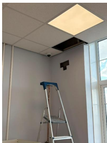
New suspended ceilings installed
