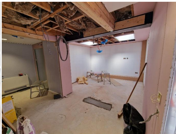
New primary classroom plastered and painted
