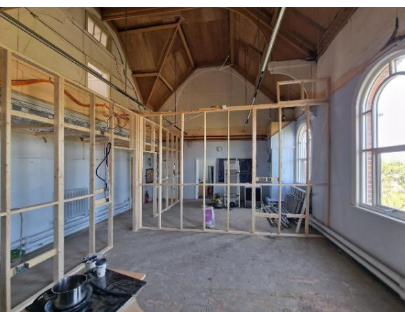
Wall partitions installed to create new Art room
