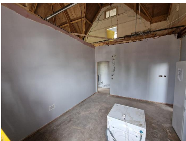
New Art room plastered and painted
