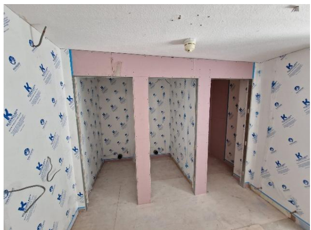
New Secondary toilet works beginning
