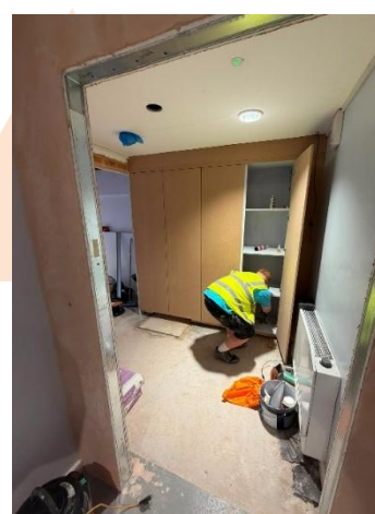
New storage area in Primary area
